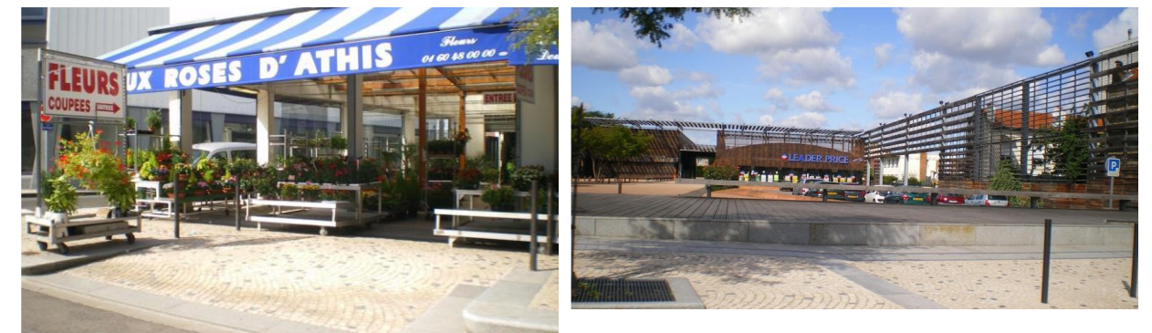
Figure 169 – Aménagements urbains (Athis-Mons)
