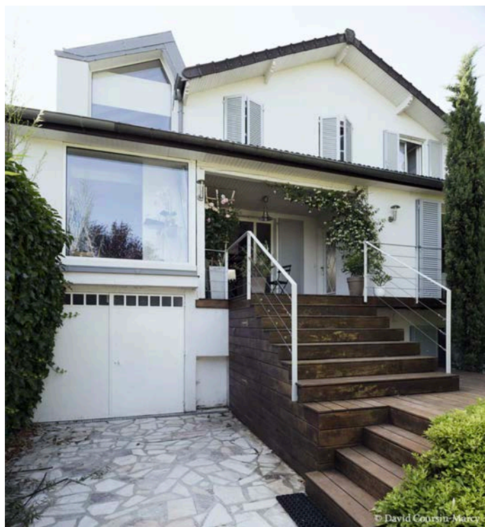
Extension maison ANGELES DUQUE - MIA ARCHITECTES
