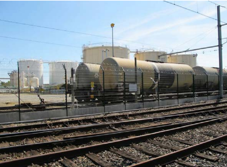
Site TOTAL Raffinage Marketing de Lospinasse (source Systra)
