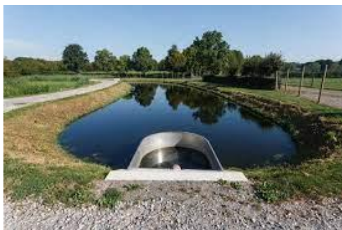
Figure 9 - Illustration bassins lagunage aéré
